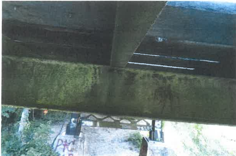
Typical condition of floor beams.
