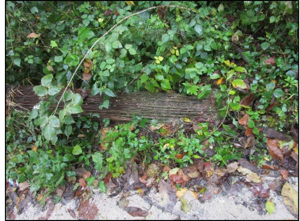
Southwest Main Cable Anchor at Grade
