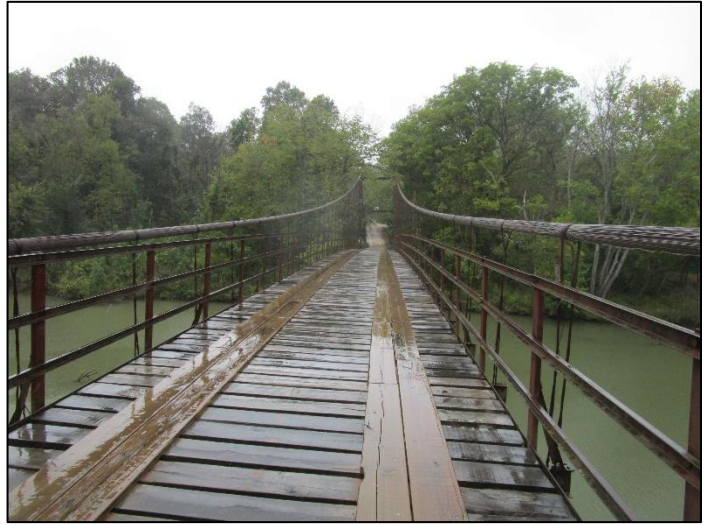
Miller Co Bridge No. 2740017
