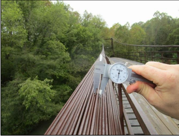
Main Cable 0.15" Diameter Wires
