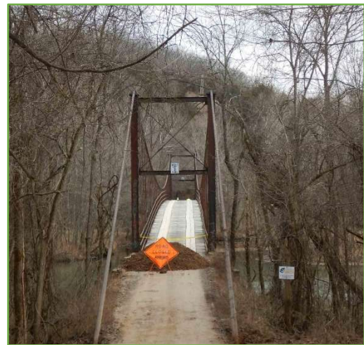
Figure 1 – Narrow unpaved approach to historic Grand Auglaize swinging bridge. (MoDOT photo)
